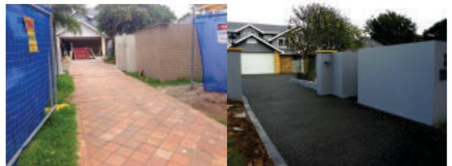
The majority of StoneSet applications involve an overlay topping or 'concrete resurfacing'. This is both economical and environmentally beneficial as the existing concrete base is not removed and sent to landfill.
